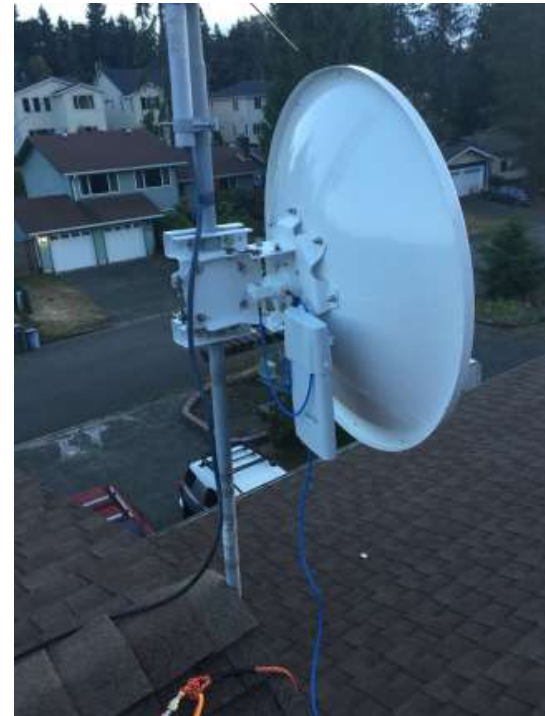
HamWAN Client Antenna
